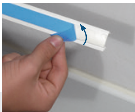
1 Simply remove the protective strip from the adhesive foam on the back of the min-trunking.
