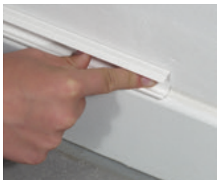
1 Position the mini-trunking against the wall.
