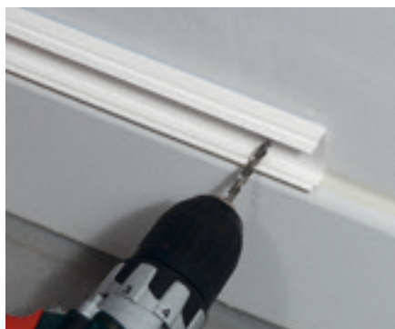
2 Attach the mini-trunking according to the composition of the wall, either nailing or screwing it on.
